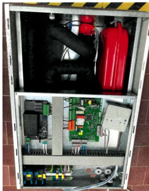
Heat pump AWM1501.090.XB12.H00.C11 - indoor unit – Without cover –
