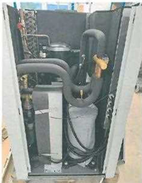
Heat pump NEXUS M17 PRO - outdoor unit - Without cover -
