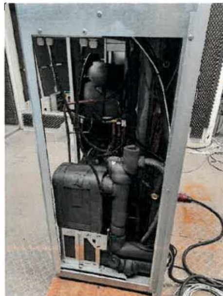
Heat pump Airadapt 4-20 - outdoor unit – Without cover –
