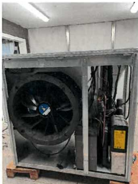
Heat pump Airadapt 4-20 - outdoor unit – Without cover –
