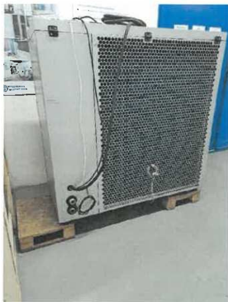
Heat pump Kolton Airadapt 4-20 - outdoor unit – Front view –
