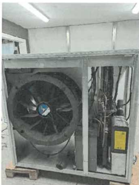
Heat pump Kolton Airadapt 4-20 - outdoor unit – Without cover –
