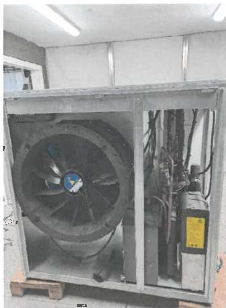
Heat pump AirAdapt 4-20 - outdoor unit – Without cover –
