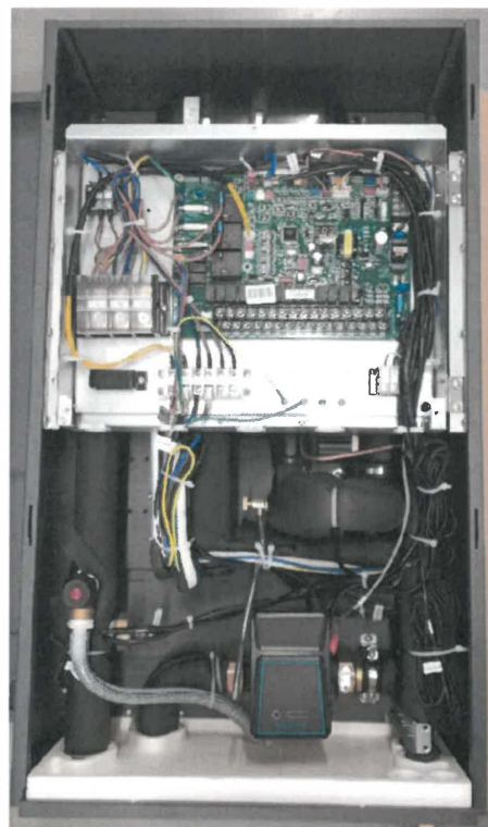
Heat pump VDS-100W/EN8BP+VDS-100B/EN8BP – indoor unit – Without cover –
