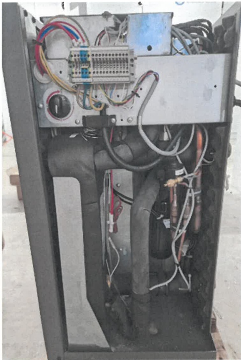
Heat pump EUROS ATMO 7 – outdoor unit – Without cover –
