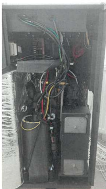
Heat pump PC-CE-MB-HT-3P-12-01 – outdoor unit – Without cover –
