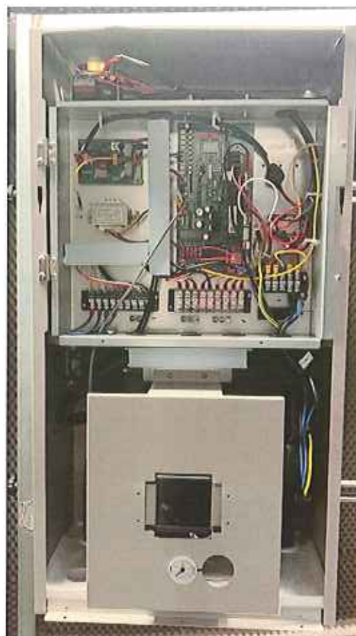
Heat pump HYDRONIC-12KW – indoor unit – Without cover –
