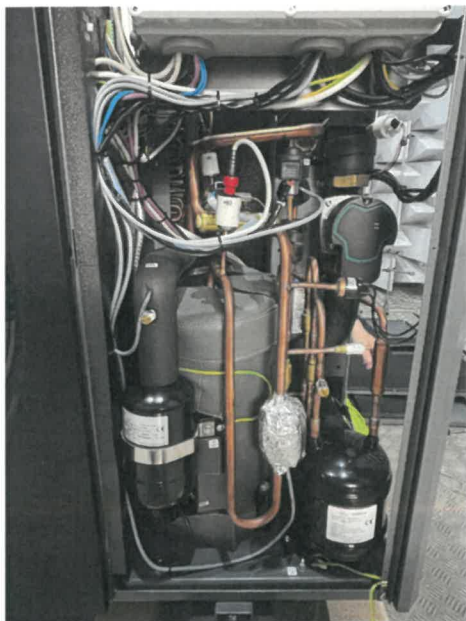
Heat pump ZHHH-P1-010K-R290-R5-M – Without cover –
