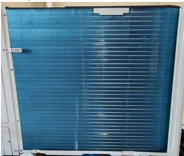
Verdampfer (Evaporator)
