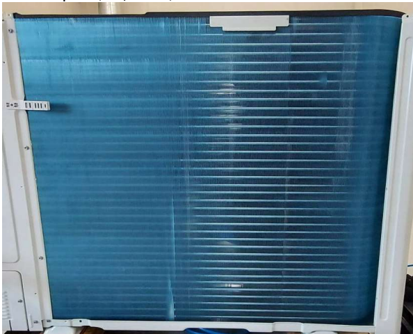
Verdampfer (Evaporator)
