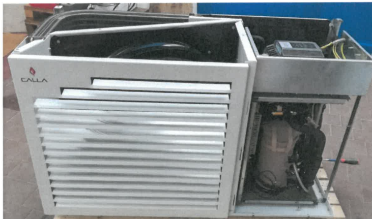
Heat pump Rakoczy 9 Monoblok – Unit without cover –
