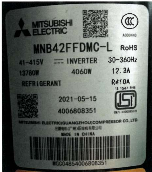
Heat pump AWM1501.090.XB17.H00.C13 - outdoor unit - Compressor label -
