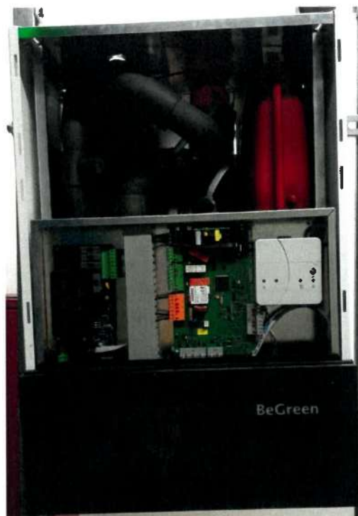
Heat pump AWM1501.090.XB17.H00.C13 - indoor unit – Without cover –
