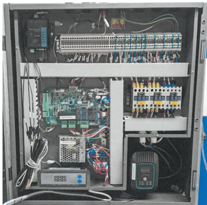
Heat pump Neoheat Eko Mono 15 (R290) – indoor unit – Without cover –
