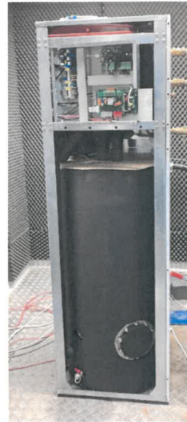
Heat pump AWM1752.075.XS10.A00.C13 indoor unit – Without cover –
