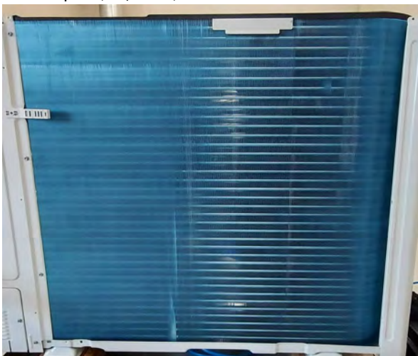
Verdampfer (Evaporator)
