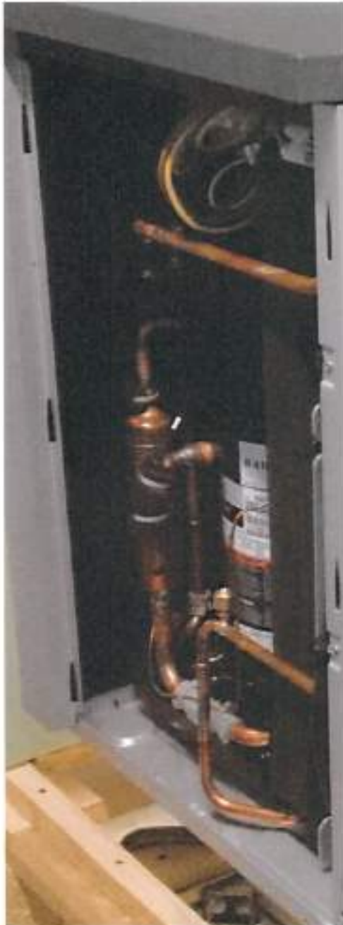
Figure 2: Refrigeration circuit
