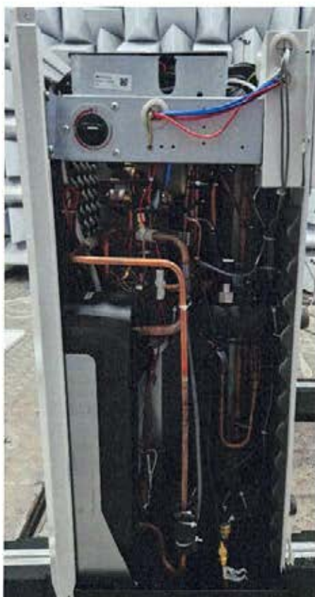
Heat pump HPOM011Z0C – outdoor unit – Without cover –
