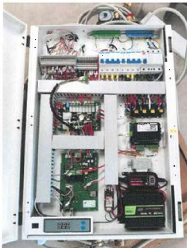
Indoor hydro-box unit HPOM020W6A – Front view without cover: Electrical part /on left/, Hydraulic part /on right/ –
