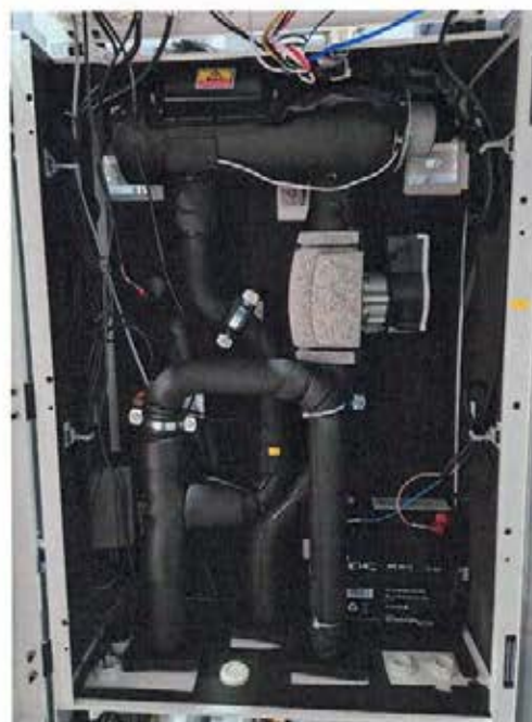
Heat pump HPOM020W6C – indoor unit – Without cover –
