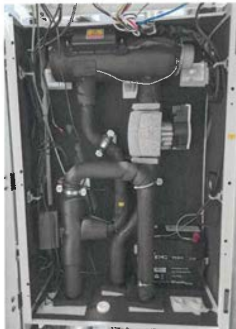
Heat pump HPOM020W6C – indoor unit – Without cover –
