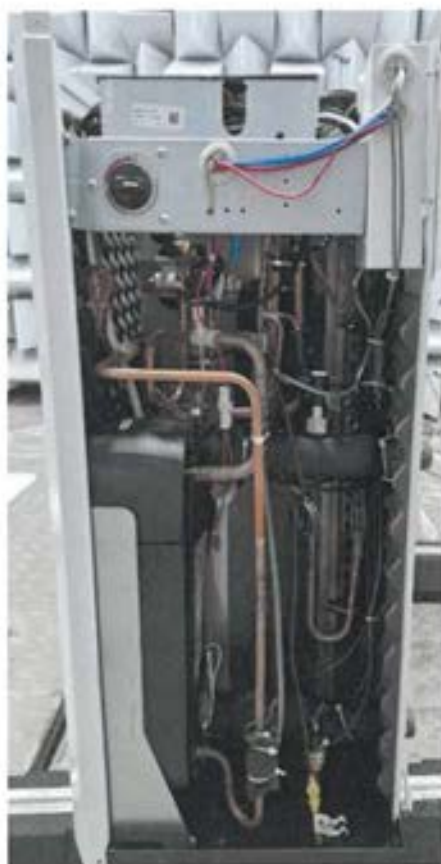
Heat pump HPOM011Z0C – outdoor unit – Without cover –
