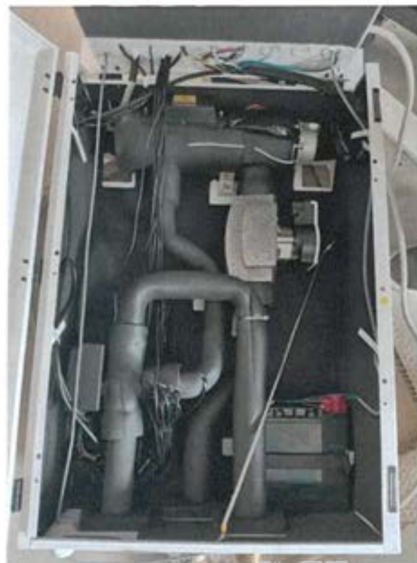
Indoor hydro-box unit HPOM020W6A – Front view without cover: Electrical part /on left/, Hydraulic part /on right/ –
