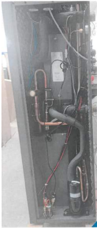
Heat pump EUROS ATMO15 – outdoor unit – Without cover –
