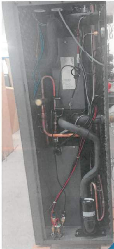
Heat pump EUROS ATMO 15 OUT – outdoor unit – Without cover –
