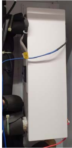
Expansionsventil (expansion valve)
