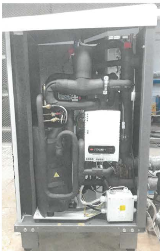
Heat pump x-change dynamic pro ac 10 AW E – Outdoor unit (without cover) –
