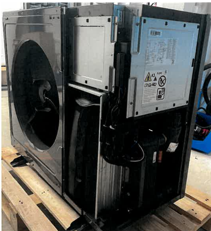
Heat pump AE080CXYDGK/EU – outdoor unit – Without cover –
