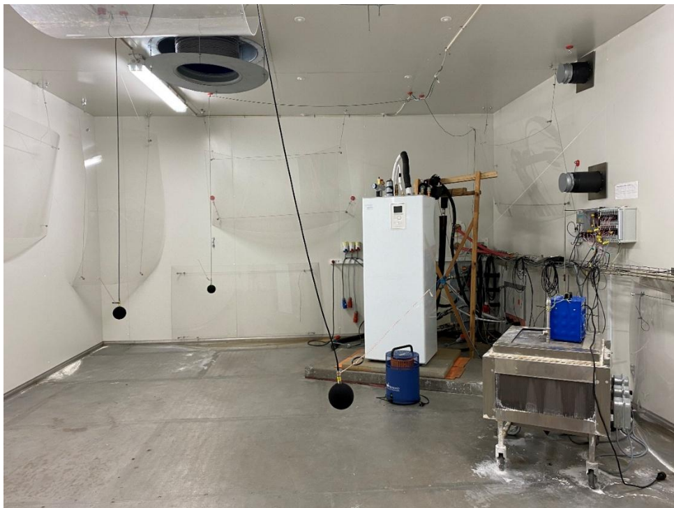
Figure 1: Indoor unit during test.
