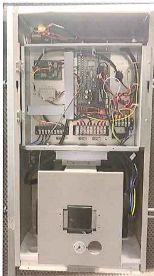
Heat pump Tivano split 12kW – indoor unit – Without cover –
