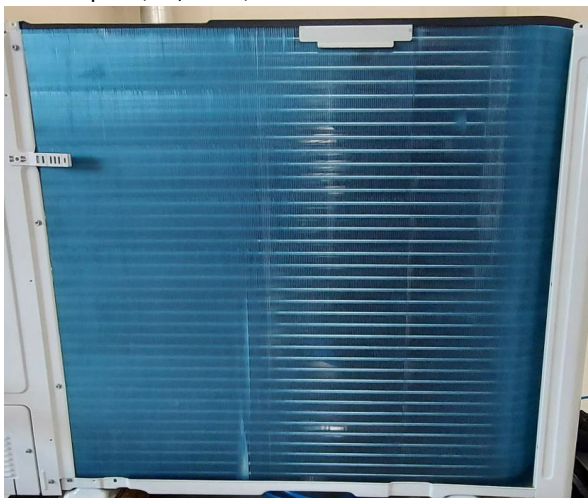
Verdampfer (Evaporator)
